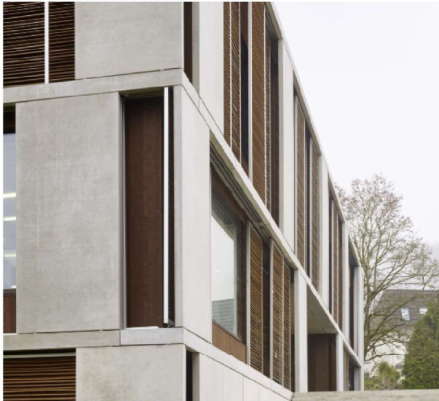
Concrete panels with inset glazing
