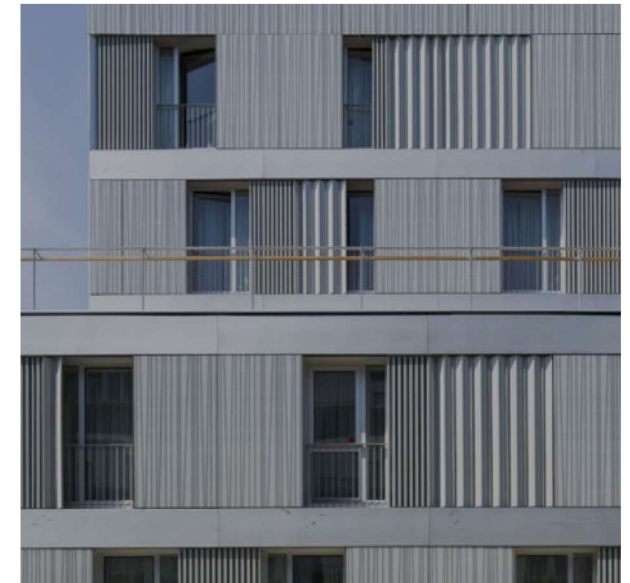
Mixed Smooth and Textured Concrete
